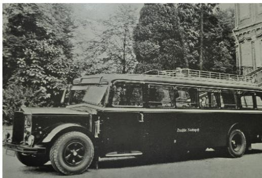
1935- Mercedes-Benz O-4000, 110cv, motor diesel, 6cil.
